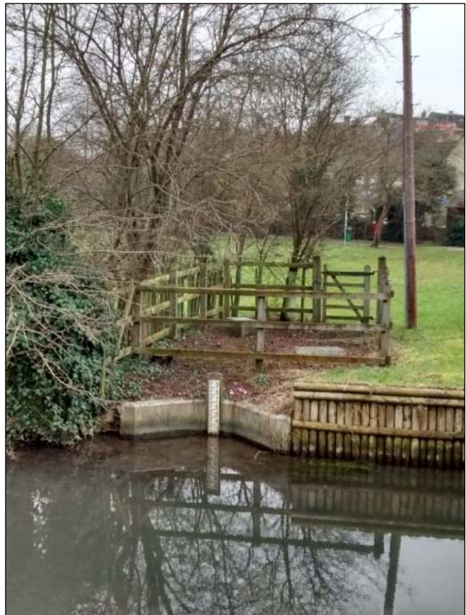
St John's Weir North Bank Sight Board with Gauging Station behind.
